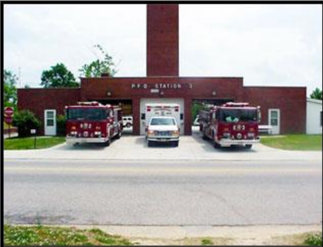
Station 3 1320 Farmer Street Petersburg, VA 23803 Built 1955
