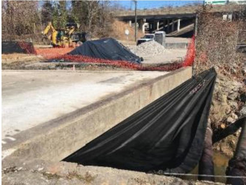
Contractor installing tarp under existing bridge deck.
