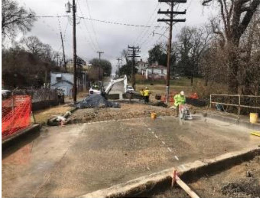
Contractor saw cutting existing bridge deck.
