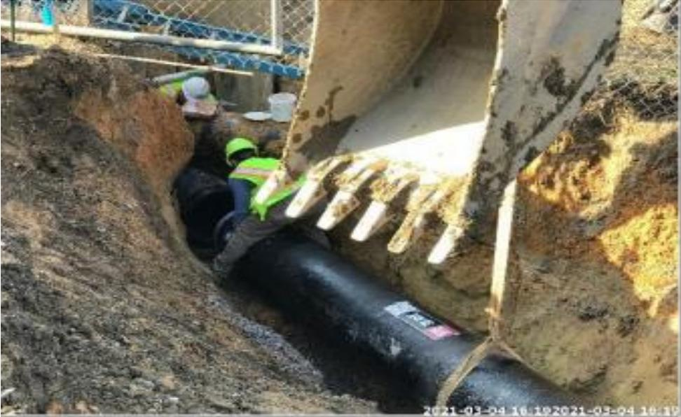
Contractor installing 18” ductile iron waterline pipe.
