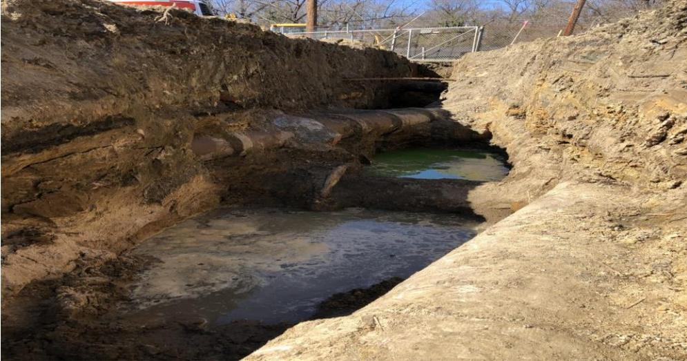
Terracotta sanitary sewer pipe and cast-iron storm sewer pipe in path of proposed location of 18” waterline.
