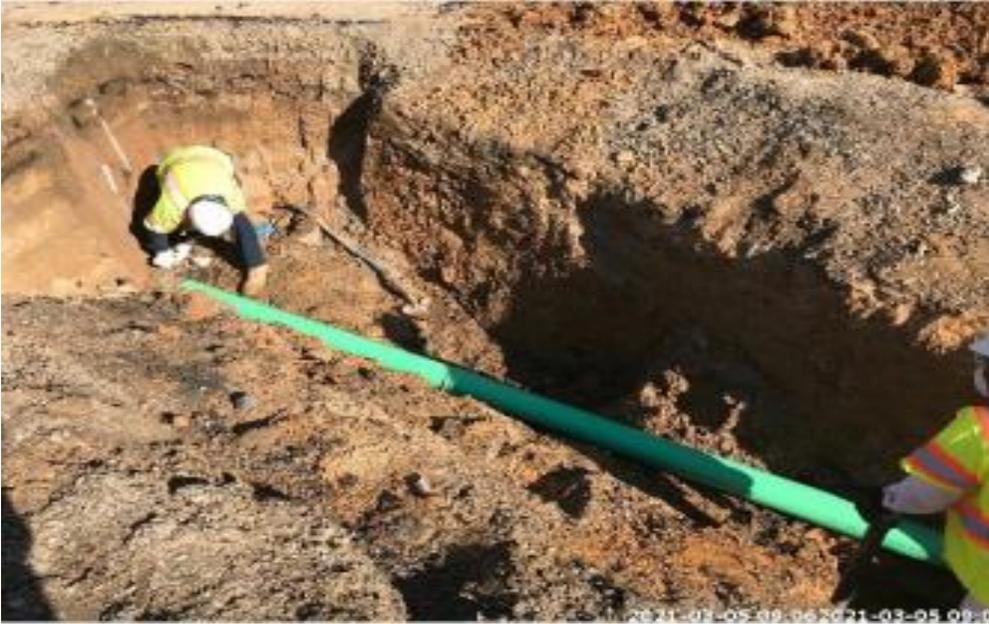
Utility Department installing 8" PVC sanitary sewer pipe.
