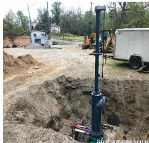
One of two line stops installed on 18" transit waterline.
