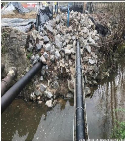
Completed 8" ductile iron waterline pipe.
